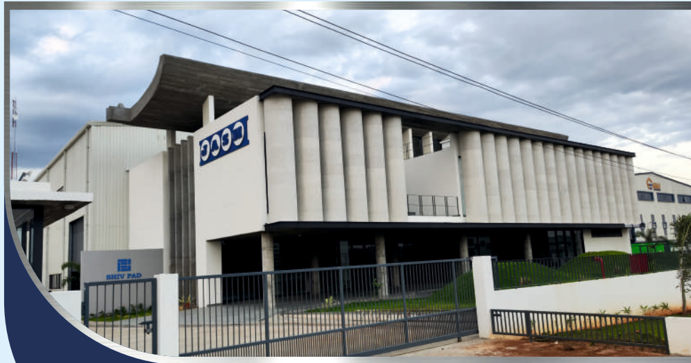
New Manufacturing facility - Vadagam Vallam, Chennai, India: In June 2026.
