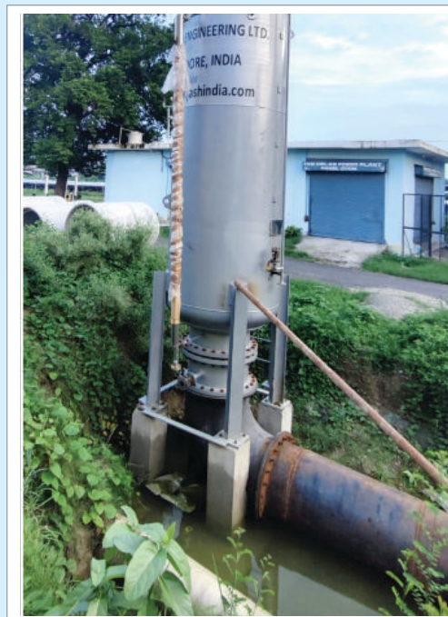
Bladder vessel 9 m3- 3nos, 1 m3-3nos supplied to Varanasi WSP project
