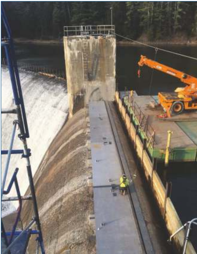
30500 x 1800 mm Structural Steel Crest Gate for Peterson Hydro Station, VT, USA
