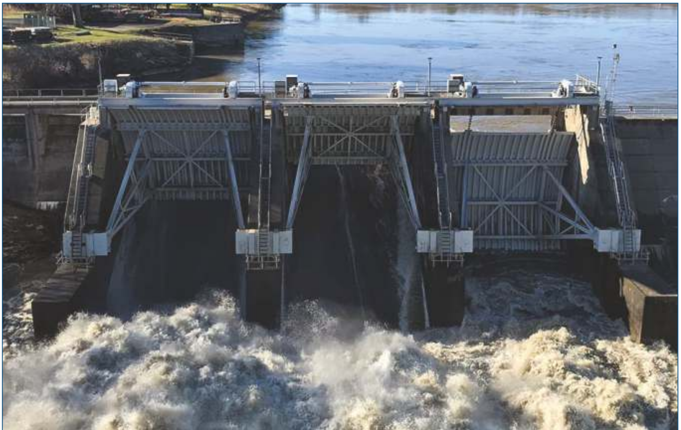
9000 x 9000 mm Structural Steel Radial Gates for Turners Falls Dam on the Connecticut River, CT, USA
