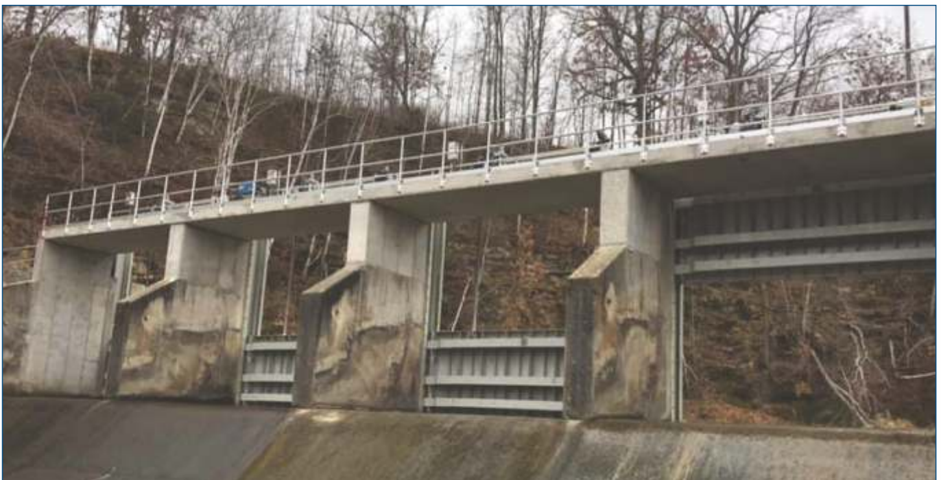
6000 x 2000 mm Structural Steel Roller Gate for Hillsboro Dam, WI, USA
