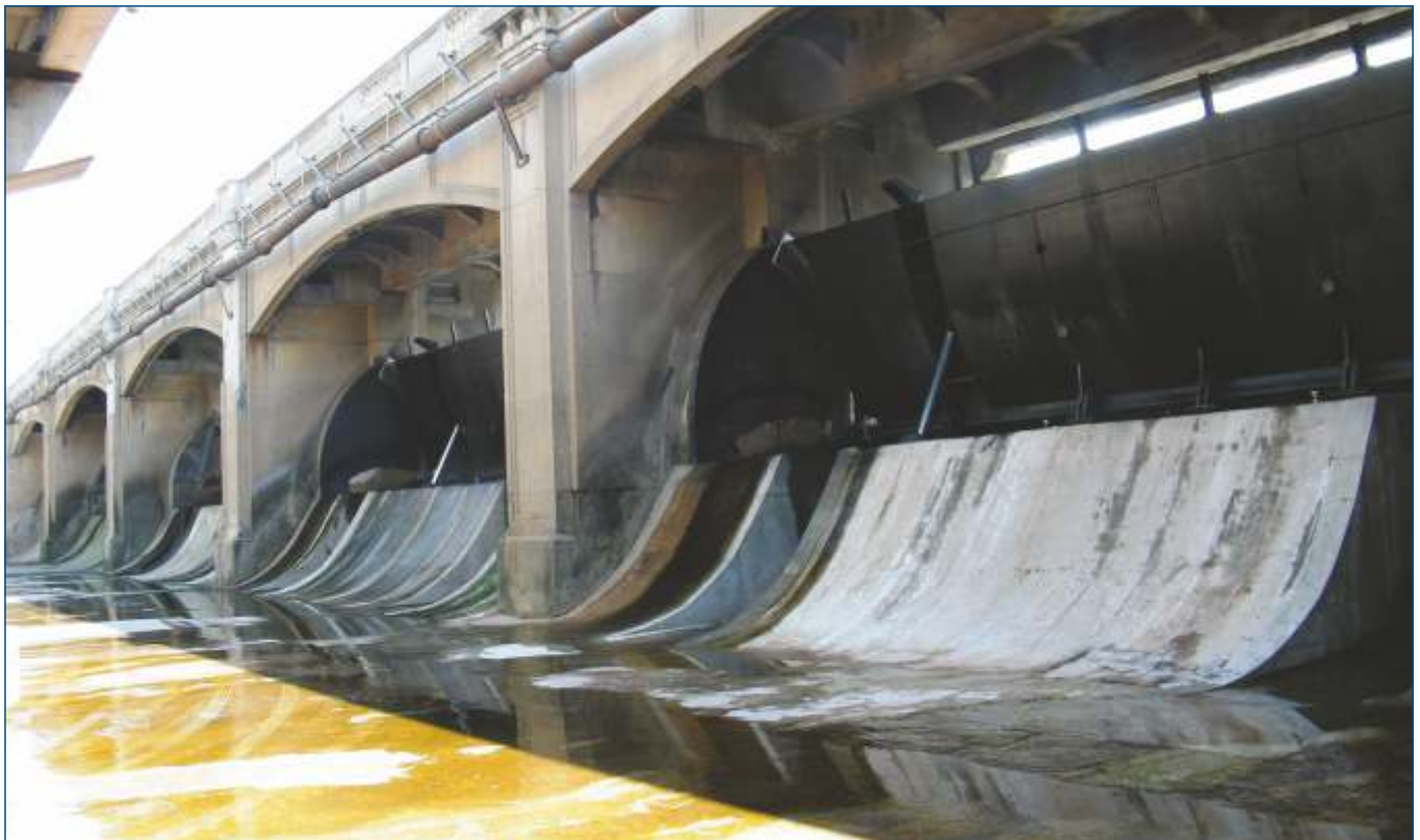
13700 x 2400 mm Structural Steel Crest Gate (Pelican Style) for Spaulding Dam, Springfield, IL, USA
