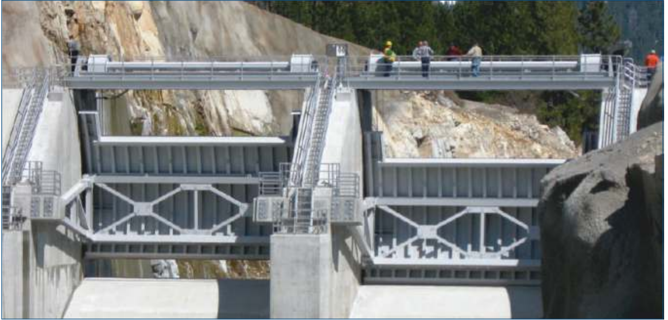
11000 x 5700 mm Structural Steel Tainter Gate for LL Anderson Dam, CA, USA
