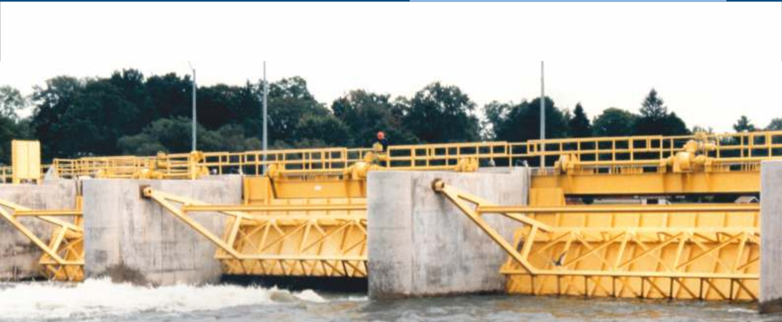
14000 x 3600 mm Structural Steel Tainter Gate for Phoenix Dam on the Oswego River, Phoenix, NY, USA
