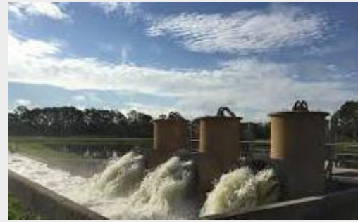
Storm water pumping stations
