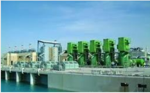
Water intake systems
