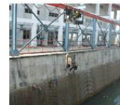
Suspended Trash Rack
