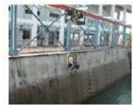
Suspended Trash Rack
