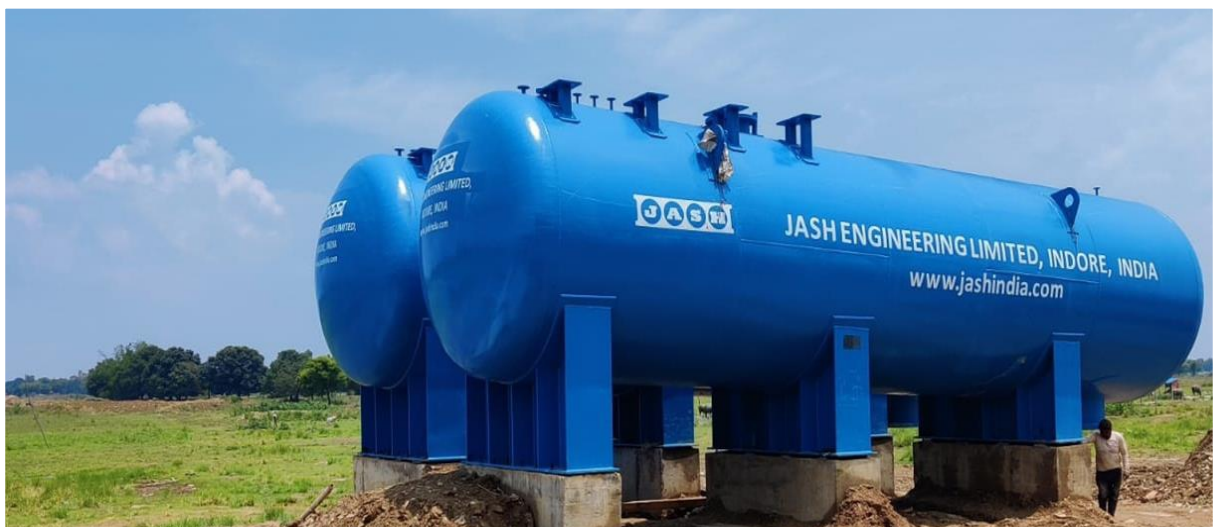
Successful Installation Of 103 M3 X 2 Air Vessels At Naigarhi -1 Project, MP
