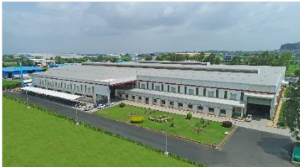
● UNIT-2 : Fabricated Products Plant
