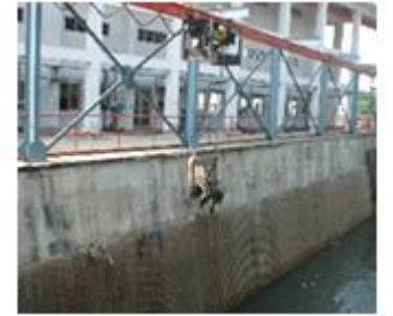
Suspended Trash Rack
