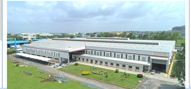
UNIT-2 FABRICATED PRODUCTS PLANT BUILT UP AREA: 155,000 Sq. ft. Turnover Capability : ₹ 175* Crore
