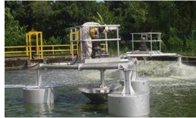
Slow speed floating aerator
