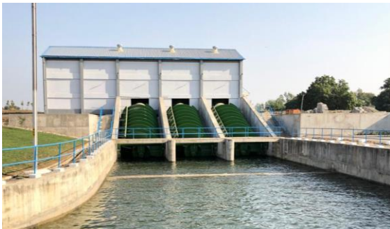
Hydropower Screw Generator
