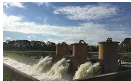
Storm water pumping stations
