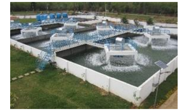
Slow speed fixed aerator
