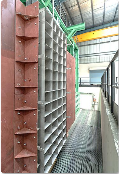
Hydro-Testing Area at Unit -4
