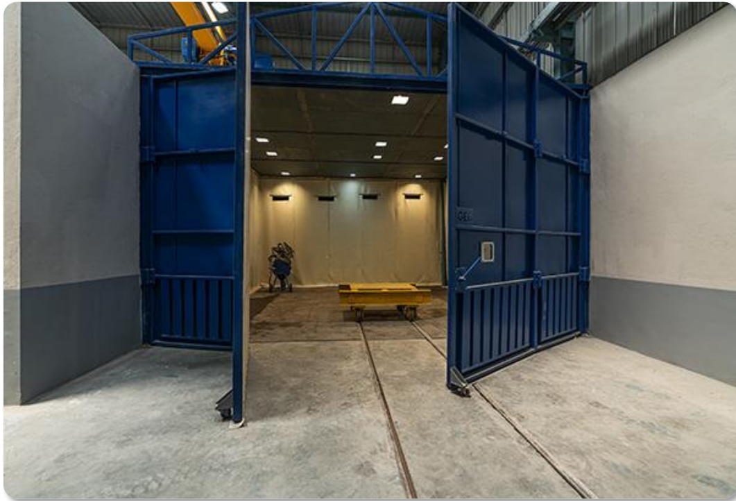
Glass Bead Blasting Area
