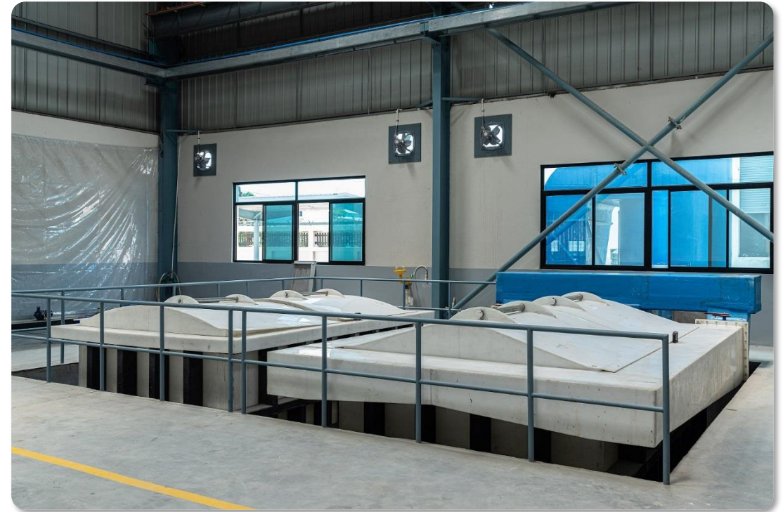
Pickling & Passivation Area
