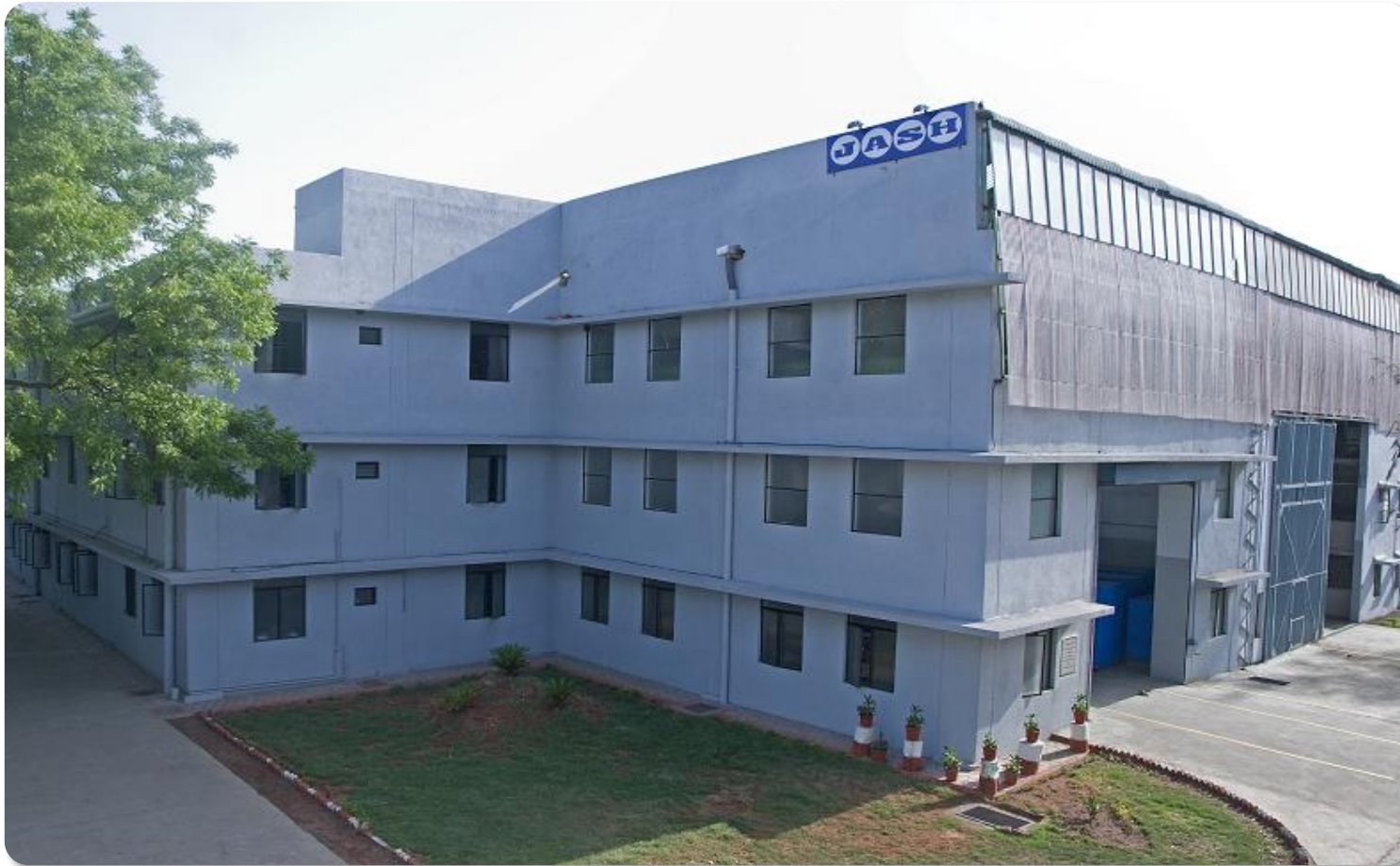
Gate Shop Outside View
