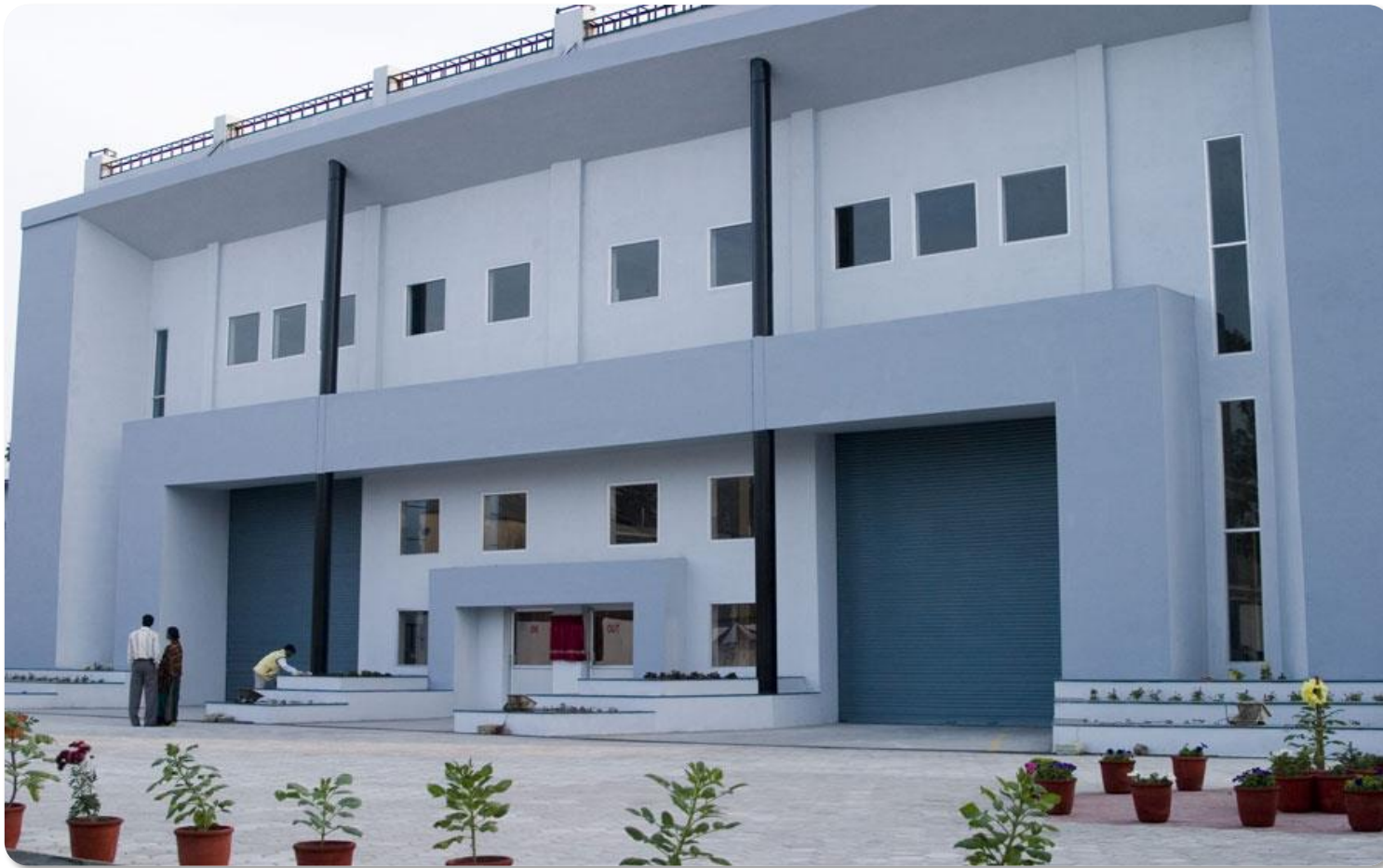
Valve Shop Outside View
