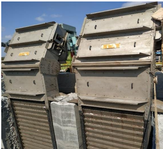
Screen after installation at Nemmeli Desalination plant, Chennai, India.
