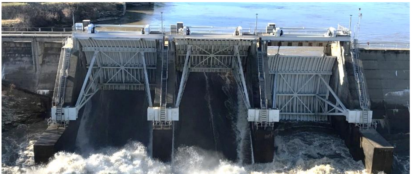
360" x 360" Structural Steel Radial Gates for Turners Falls Dam on the Connecticut River, USA
