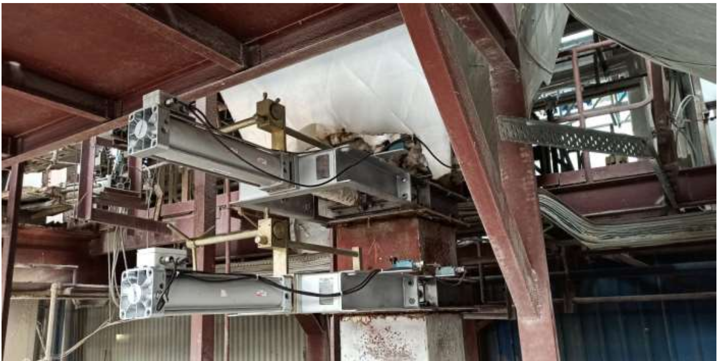
Installed Jash Fabricated Slide Gate Valve, Model VEG, Series C 531
