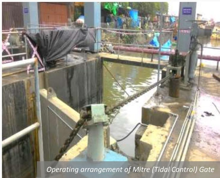
Operating arrangement of Mitre (Tidal Control) Gate
