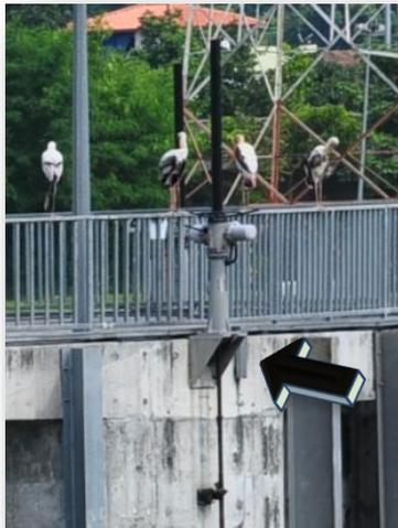
The bracket has to be designed to take the operating thrust coming from gate.
