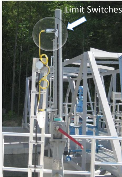
Remote indications of gate opening arrangement is provided on rising spindle gates to indicate “OPEN” or “CLOSE” position of gate at remote position in control room.
