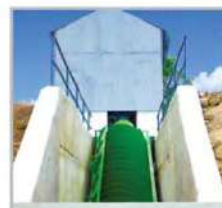
Archimedean Screw Turbine
